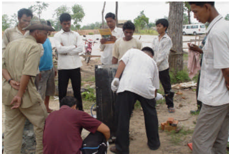
Making the first filter in Village #2
