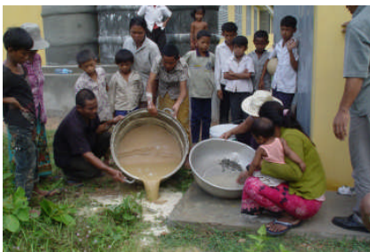
Washing the sand to put in filter
